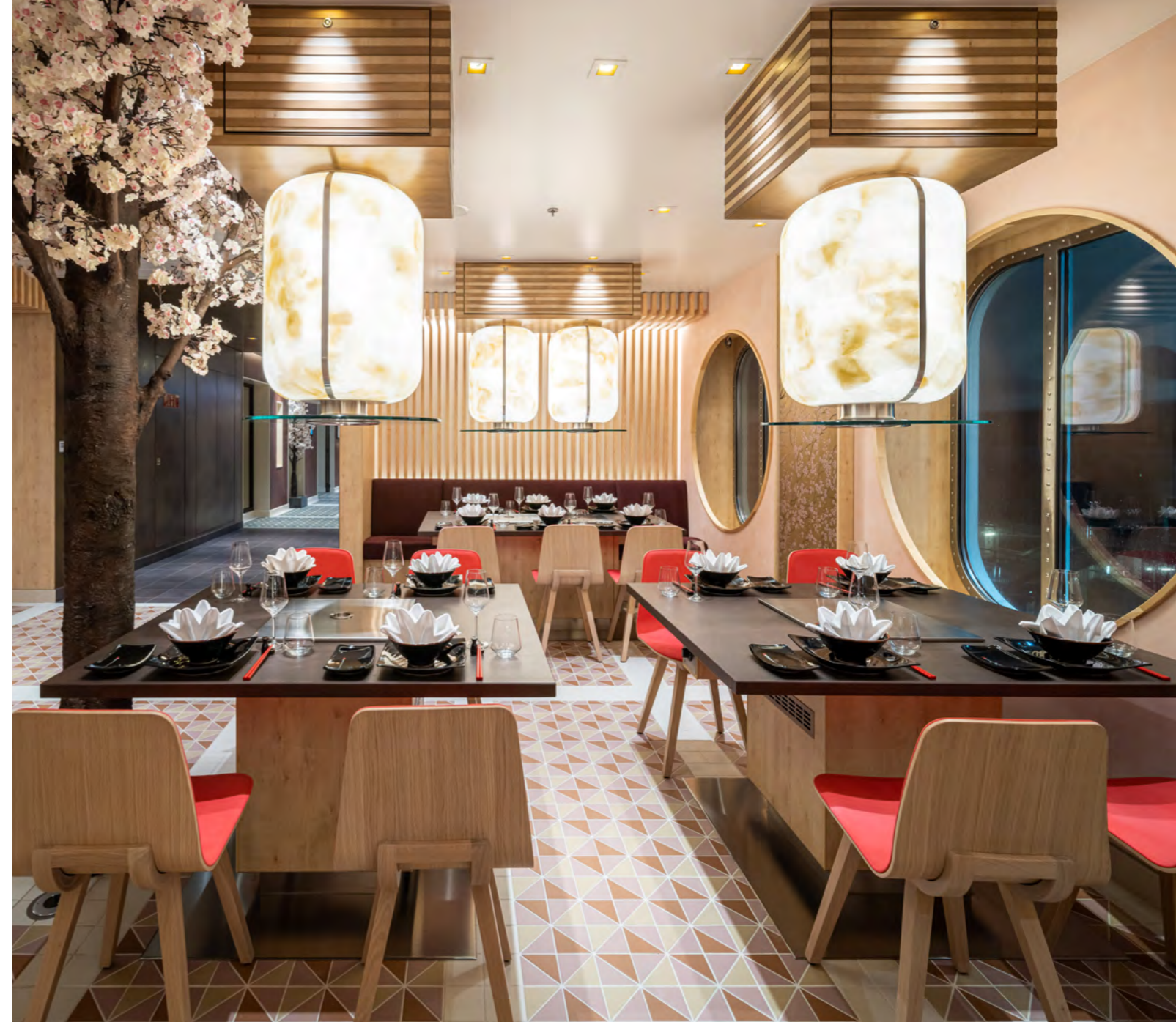
Project reference: AIDAcosma cruise ship, Sushi House, Halton's hoods installed above the tables. Photo: Alexander Rudolf.
